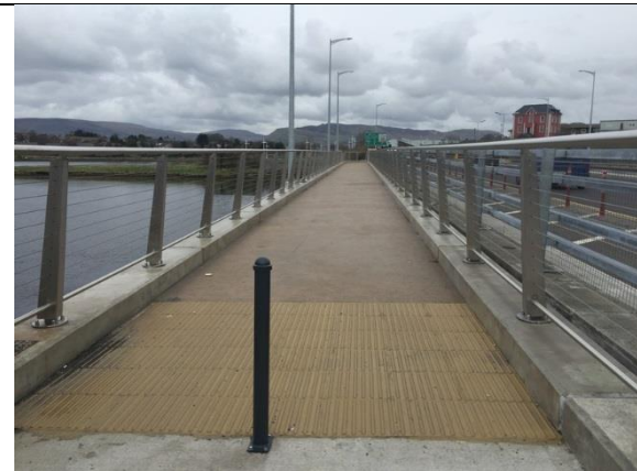
Plate 3: Recently completed upgrading / widening of Hughes Bridge
