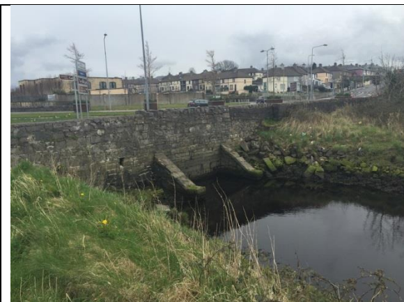
Plate 17: West (coast) face of Copper River Culvert
