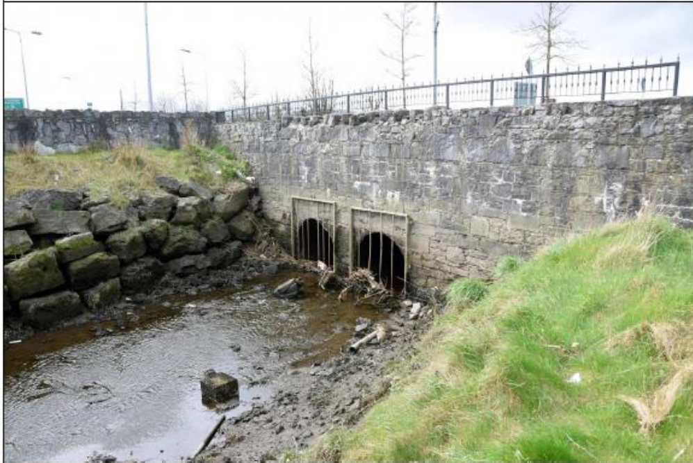
Plate 5 Upstream view of the N4 Bridge over the Copper River.
