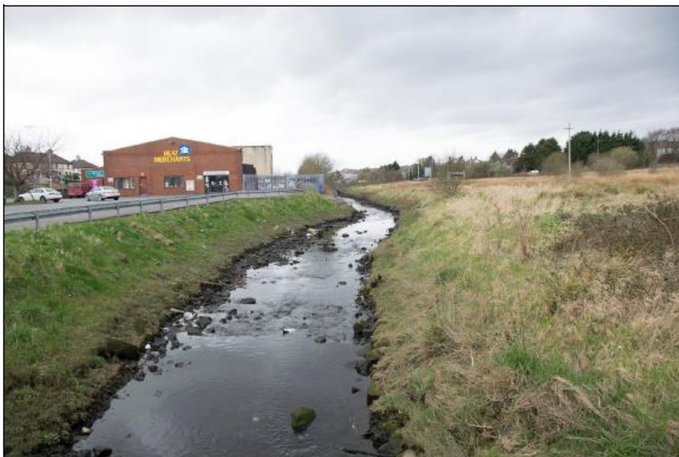
Plate 8 Copper River approximately 200m upstream of the N4 Bridge.
