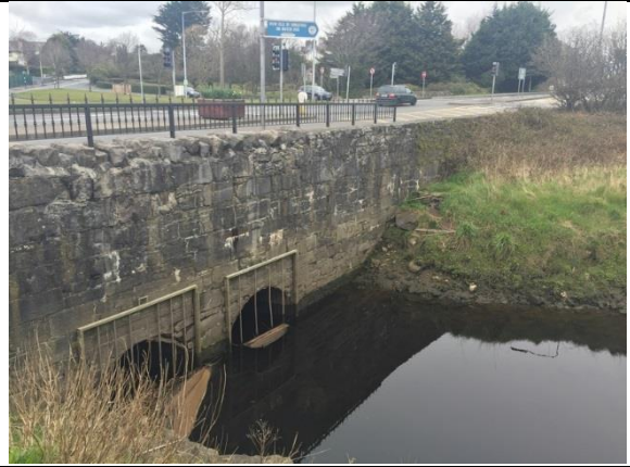
Plate 26: East face of Copper River Culvert
