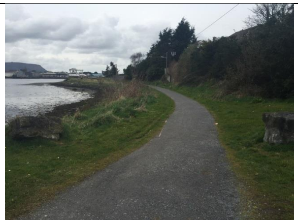
Plate 18: View west of footpath / cycleway along north side of Sligo Bay at Cartron
