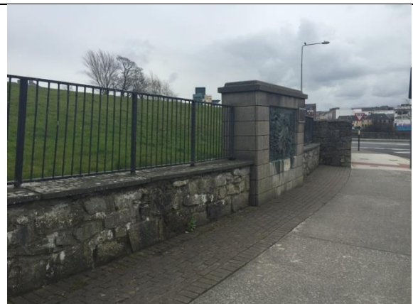
Plate 6: Feature section of wall at Constance Markievicz House with 'The Pursuit of Diarmuid and Grainne' artwork
