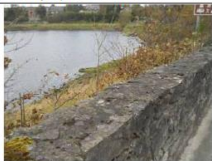
Raised wall on downstream face of N4
