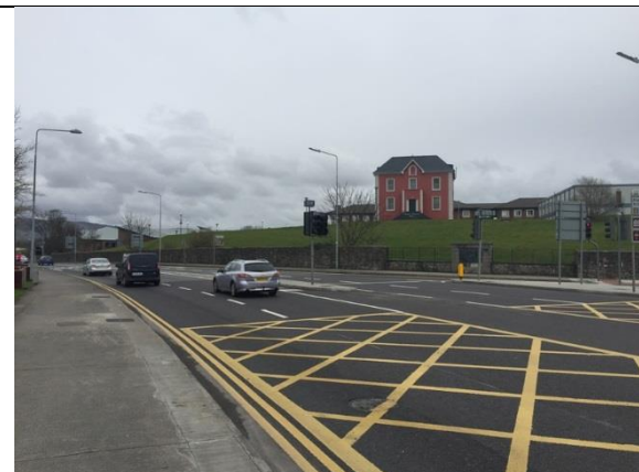
Plate 5: View north from Hughes Bridge to Constance Markievicz House
