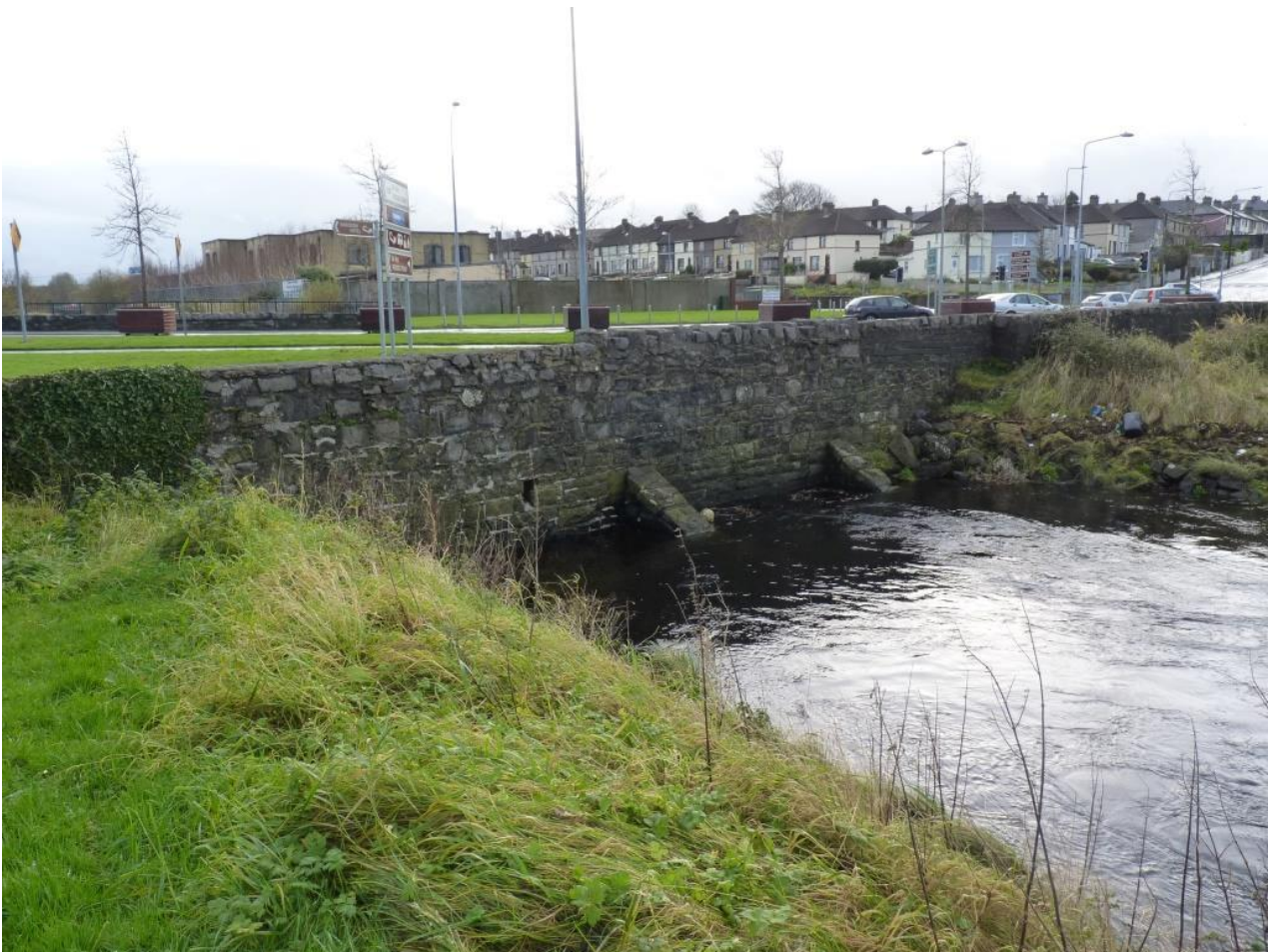
Plate 5: West elevation of the River Copper culvert (Site AH5)
