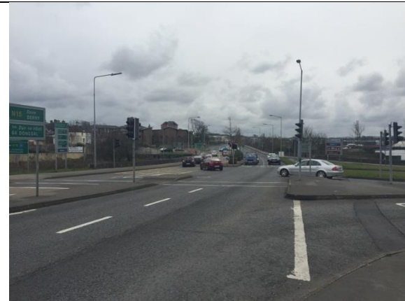
Plate 21: View south over N4/N15/N16/R291 Road Junction
